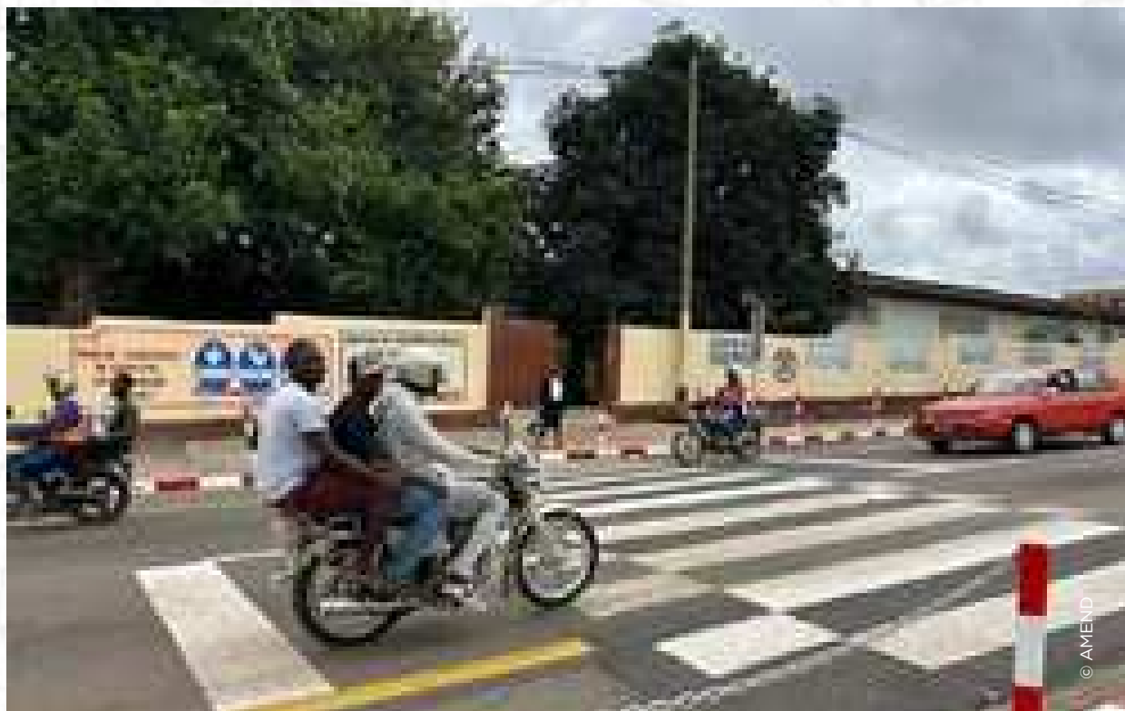
Image 65 : After the improvement of pedestrian crossings near schools.
