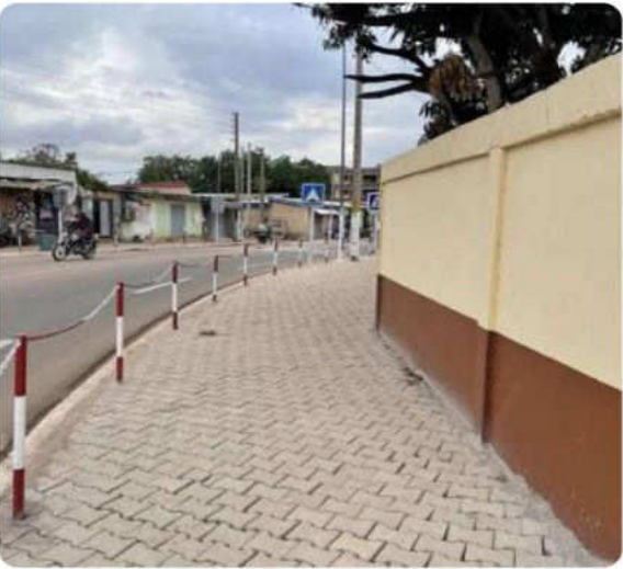
Pilot project to improve road safety around schools, Bouaké
