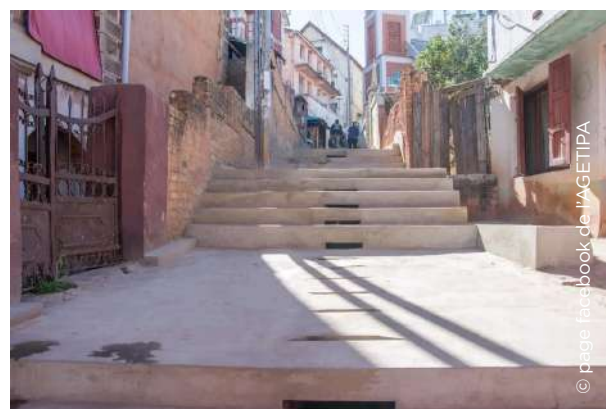
Image 34 : Construction of a staircase.
