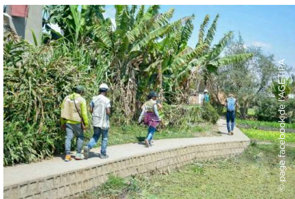
Image 33 : Construction of a footpath along the edge of an agricultural area.
