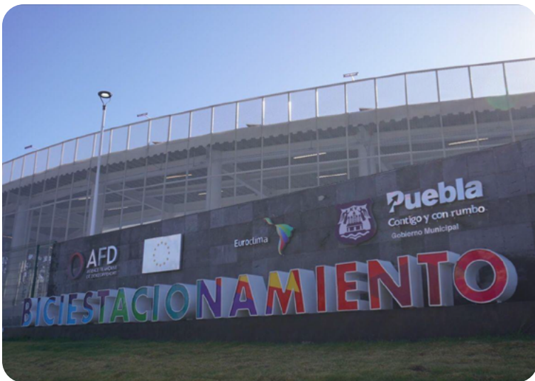
Figure 2 Bicycle parking facility at Margarita BRT terminal (Puebla, Mexico) Source: AFD (LinkedIn)
