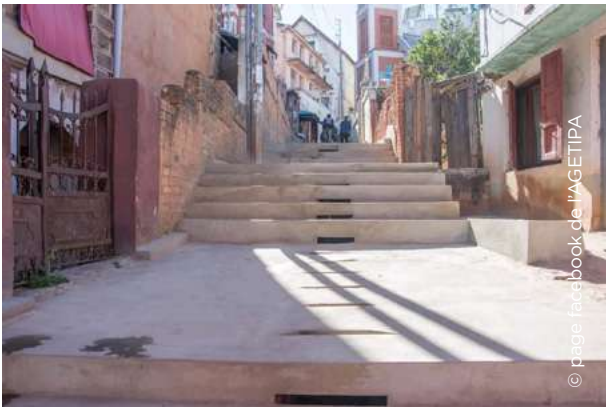
Image 34 : Construction of a staircase.
