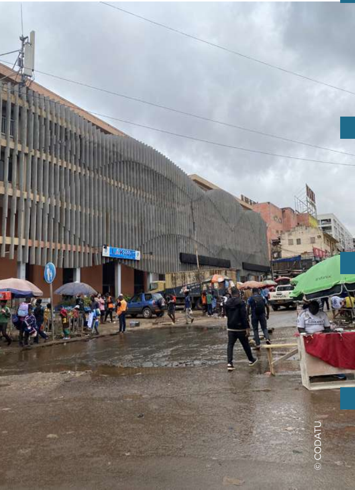
Image 48 : Pedestrians facing flooded road.
