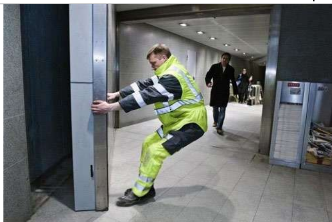
Figure 17. Flooding gates in a metro station in Copenhagen
