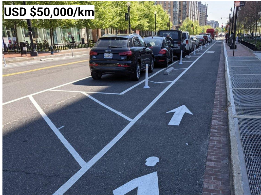
Paint and temporary materials
