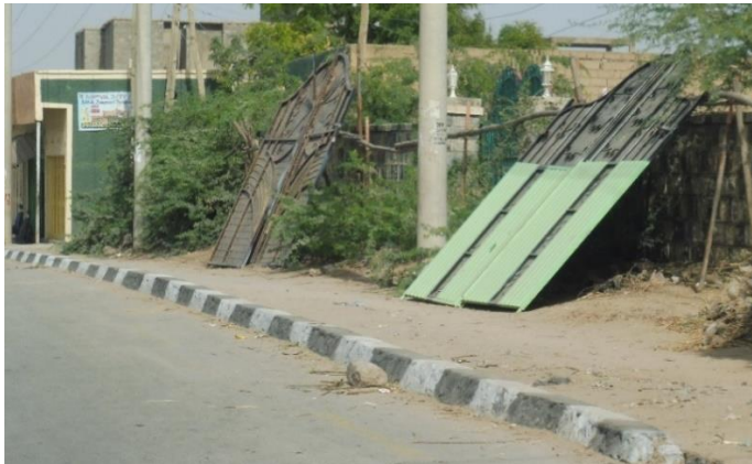
Sidewalk occupied by commercial displays, vegetation and building, thus preventing continuous pedestrian route
