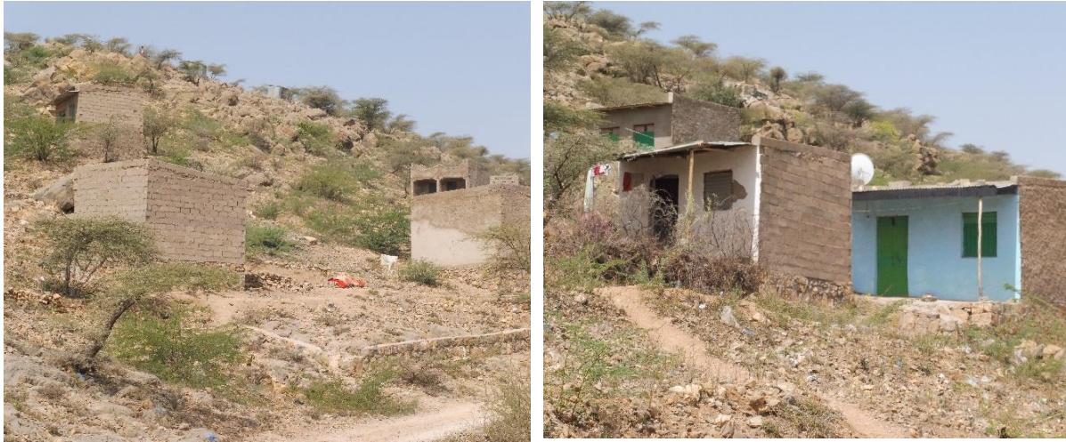
Informal dwellings scattered on the slopes overlooking Goro district under construction (left) and constructed (right). These small block houses made of cement blocks are rural types of habitat brought to the city.
