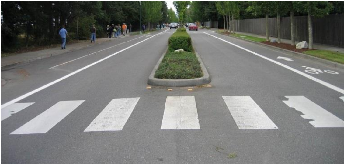
Figure 52. Raised landscaped median. Source: Designing for Pedestrian Safety
