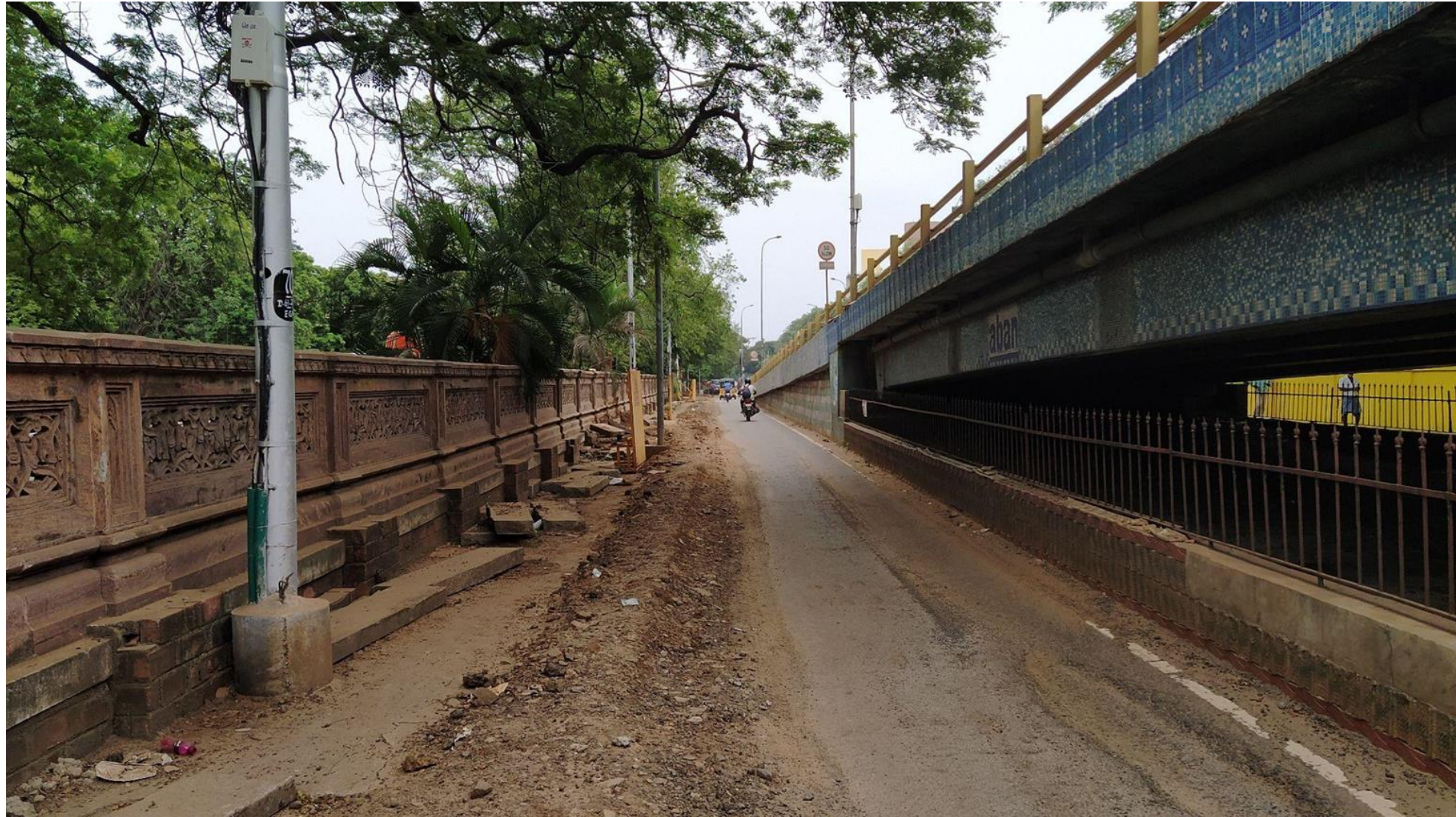
Photos: Pantheon Road, Egmore, Dug up for upgrading electricity lines | Source: ITDP India
