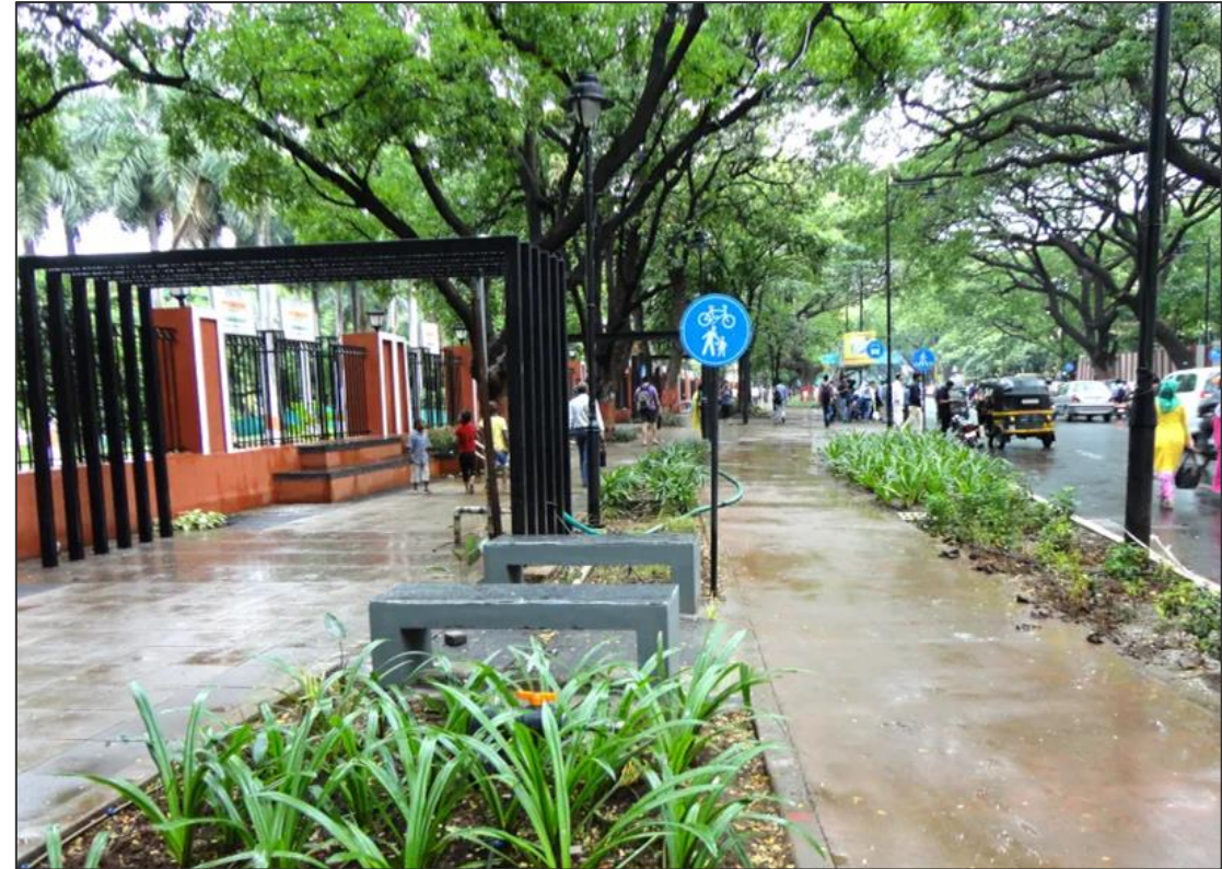
Complete street redesign and utility overhaul Source: ITDP India
