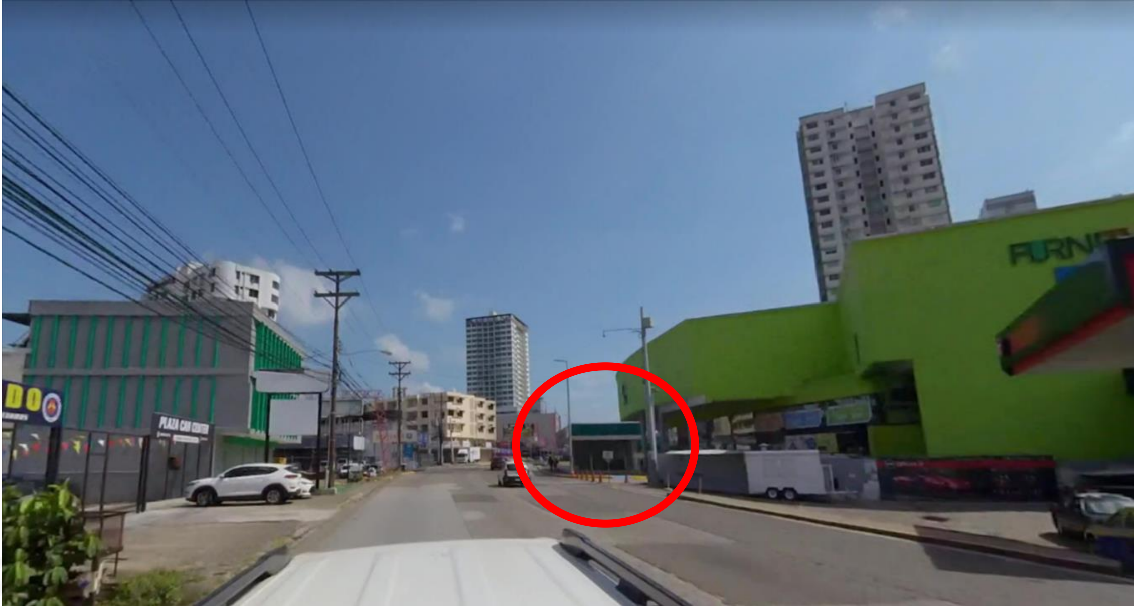
New metro station in Panama lacks usable sidewalks and cycle lane. Source Google Streetview
