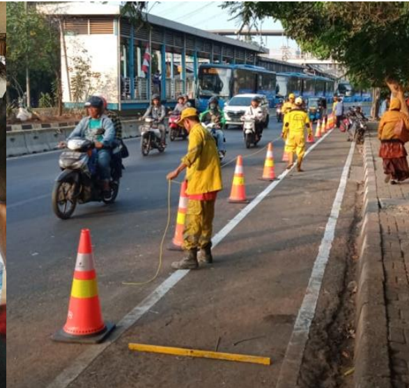
Field Installation (Source: Public Works Agency)
