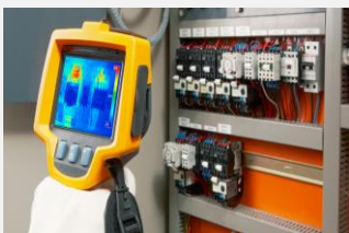
Figure 87. Example of thermographic inspection (source: Veritas Technologies Ltd.)
