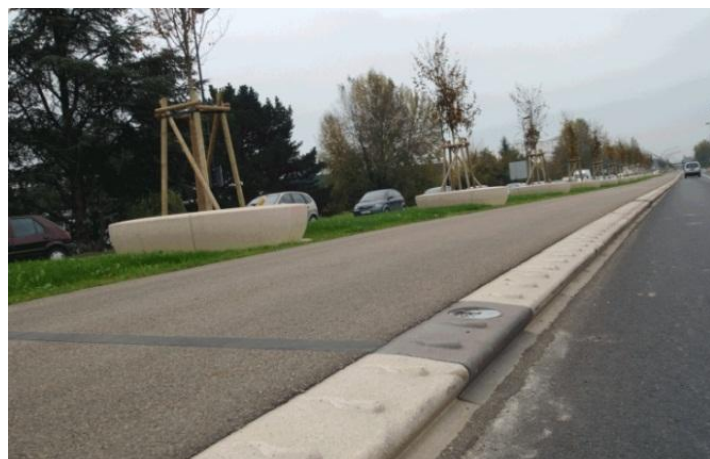
Figure 104. Elevated exclusive bus corridor in Nantes, France
