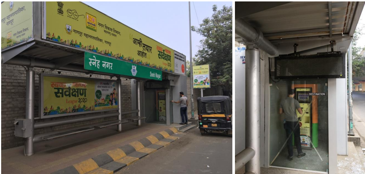
Figure 106. New Nagpur City Bus stop and Smart City Kiosk
