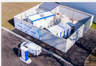
Hydrogen station filling (source: McPhy)
