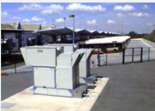
CNG plant in Poitiers, France (source: Transbus)
