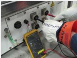
Example of electrical measurement (source: Novabus)
