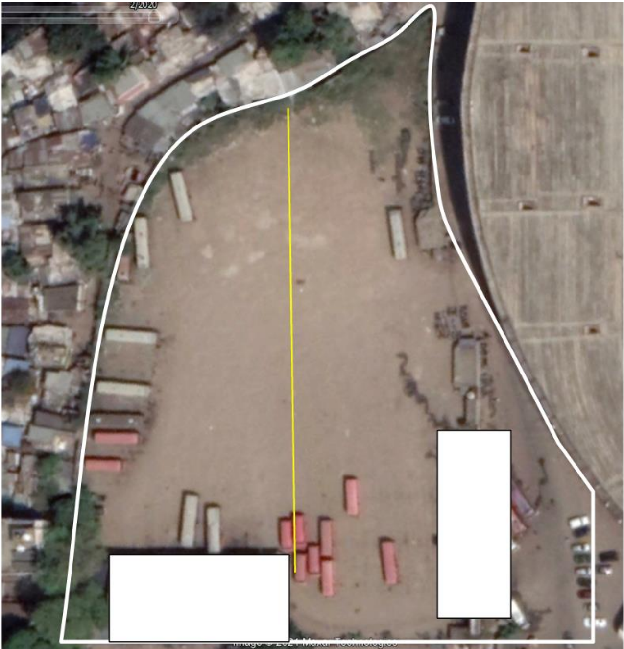
Figure 110. Aerial view - Ptwardhan 2 depot
