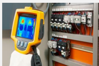
Example of thermographic inspection (source: Veritas Technologies Ltd.)
