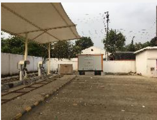
Electric bus chargers at Olectra Greentech - BYD Depot
