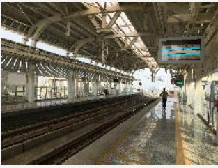
Platform at Orange Line Jaiprakash Nagar Station
