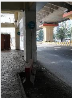
Feeder buses docking bay at Orange Line Jaiprakash Nagar Station
