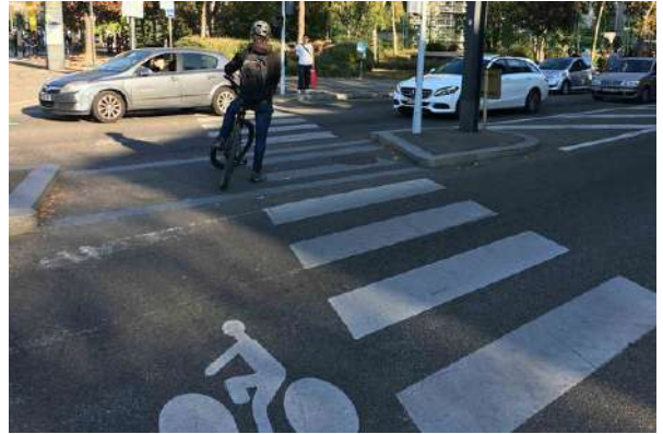
Cycle crossing with dedicated waiting space within the traffic island, Mulhouse, France
