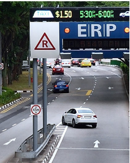
In Singapore, the congestion charge zone is delineated by overhead gantries which show the current price to enter the zone. SOURCE: Tim Adams (Flickr)
