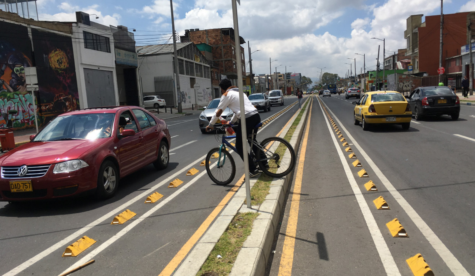
Figure 6. Cycle paths in the central lane may generate access and safety issues, example from Bogotá (Carrera 24). Photo: Carlos Felipe Pardo
