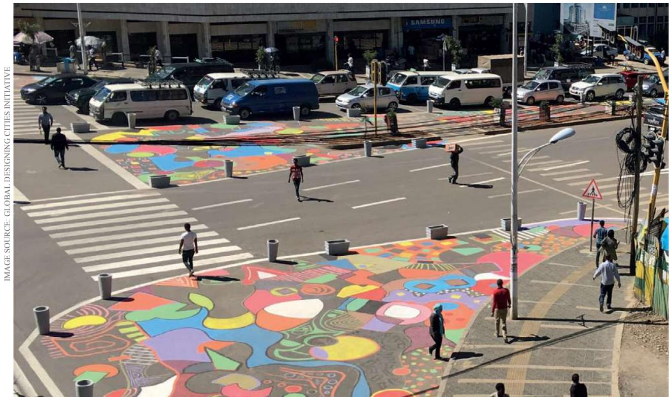
Figure 20. Pilot retrofits at Le Gare have demonstrated how reduced turning radii and crossing distances can improve pedestrian safety.
