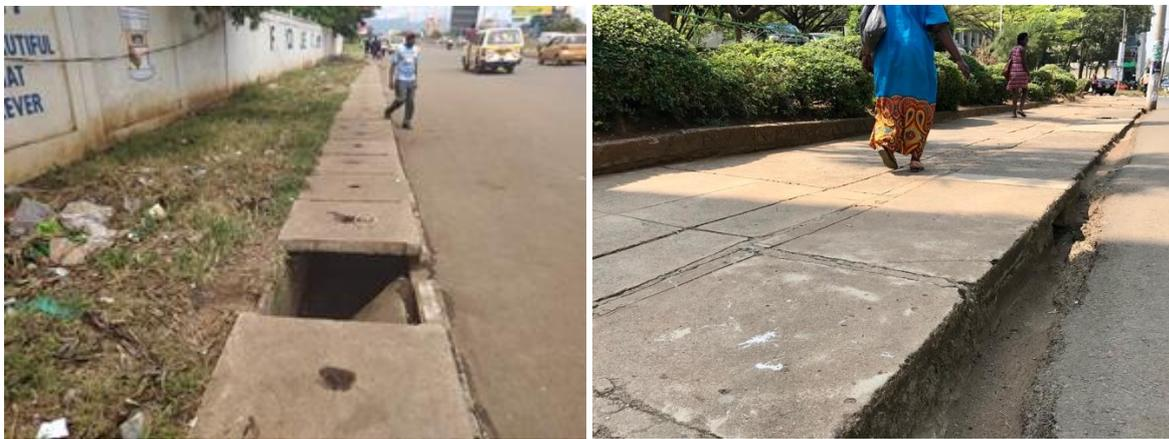
Figure 86: Loose drain covers make for a poor walking surface (left). A well-finished footpath on top of a major stormwater drain provides a comfortable walking surface (right).
