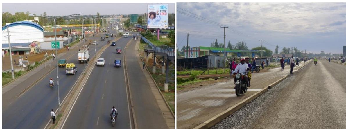
**Figure 55: While service lanes on Nairobi Rd sometimes function as shared spaces, most stretches lack traffic calming elements that would make them safe for walking.**
