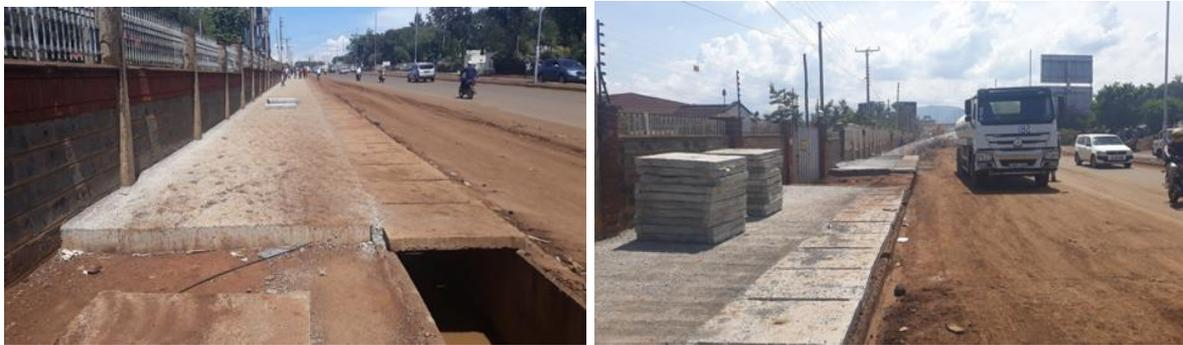
Figure 56: The Kenyatta Highway project includes concrete footpaths along some stretches. However, the design does not incorporate universal access features or tree cover.
