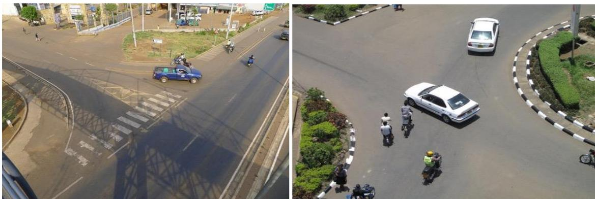
Figure 18: Wide turning radii at intersections encourage speeding by vehicles, thus making it unsafe for pedestrians to cross the road.
