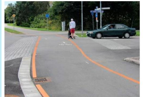
Junction with continuous cycle lane
