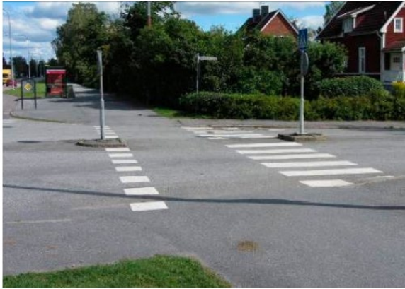
Junction before being rebuilt
