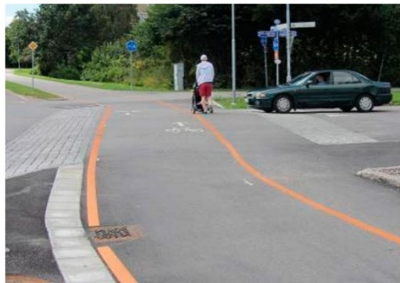
Junction with continuous cycle lane
